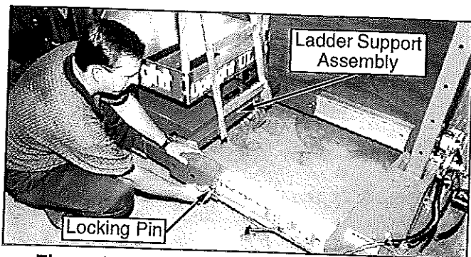
Figure 7: Installing the Ladder Assembly
